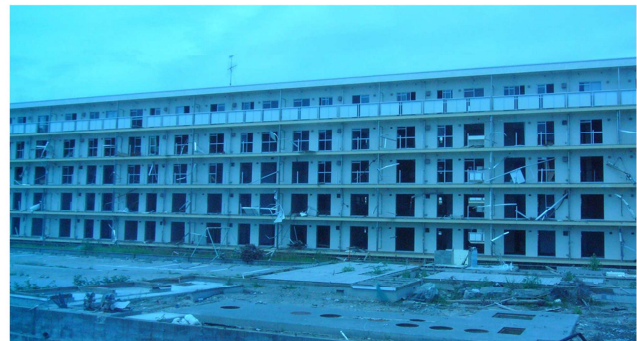
Ohfunato city, fifth stage mansion completely damaged upto 4th floor
