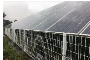
(不適切な柵塀設置の事例)
